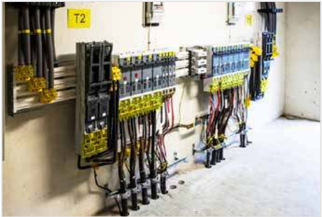
Examples of using Kabeldon products on the wall in low voltage switchgear, Sweden.
